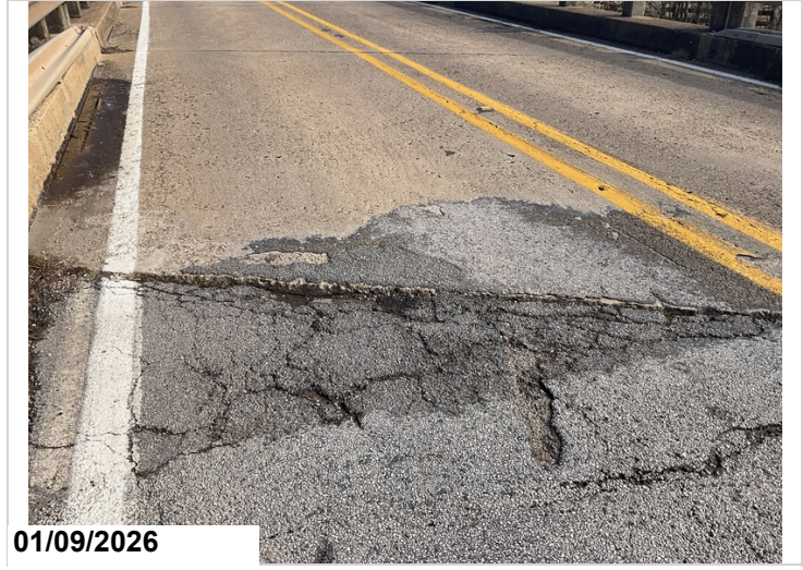
Approach leveling needed at the beginning left lane.
