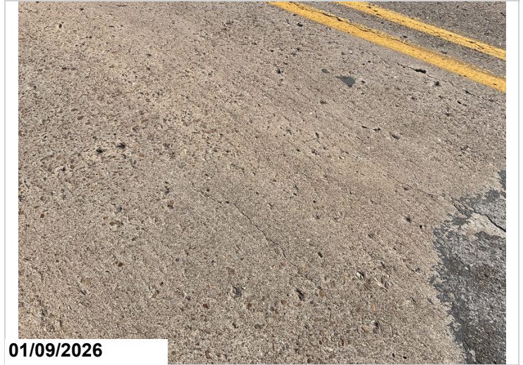
Unsealed cracking in the deck.
