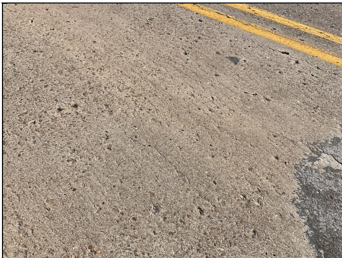
Unsealed cracking in the deck.
