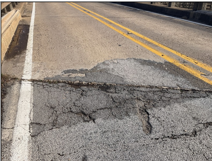
Approach leveling needed at the beginning left lane.
