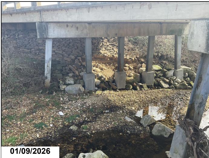
Area of rip rap displacement at the abutment #2 slope. 8' by 23' long.
