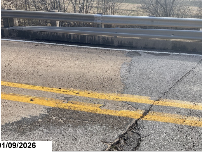
Typical asphalt patched areas in the deck.
